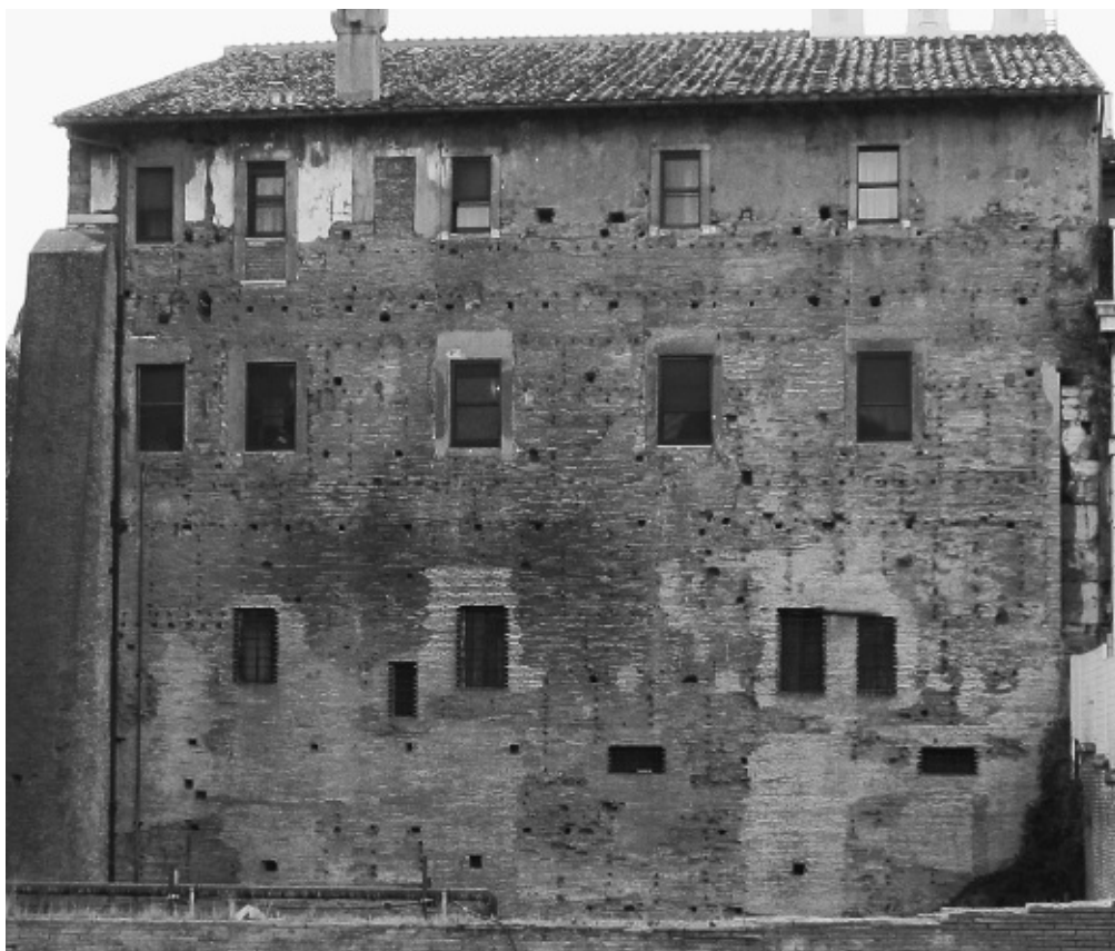
FIGURE 6.6 The wall on which the marble plan of Rome was originally mounted. Note the holes for the clamps which kept the slabs in place. Photograph by Elizabeth Robinson, reproduced with permission.
